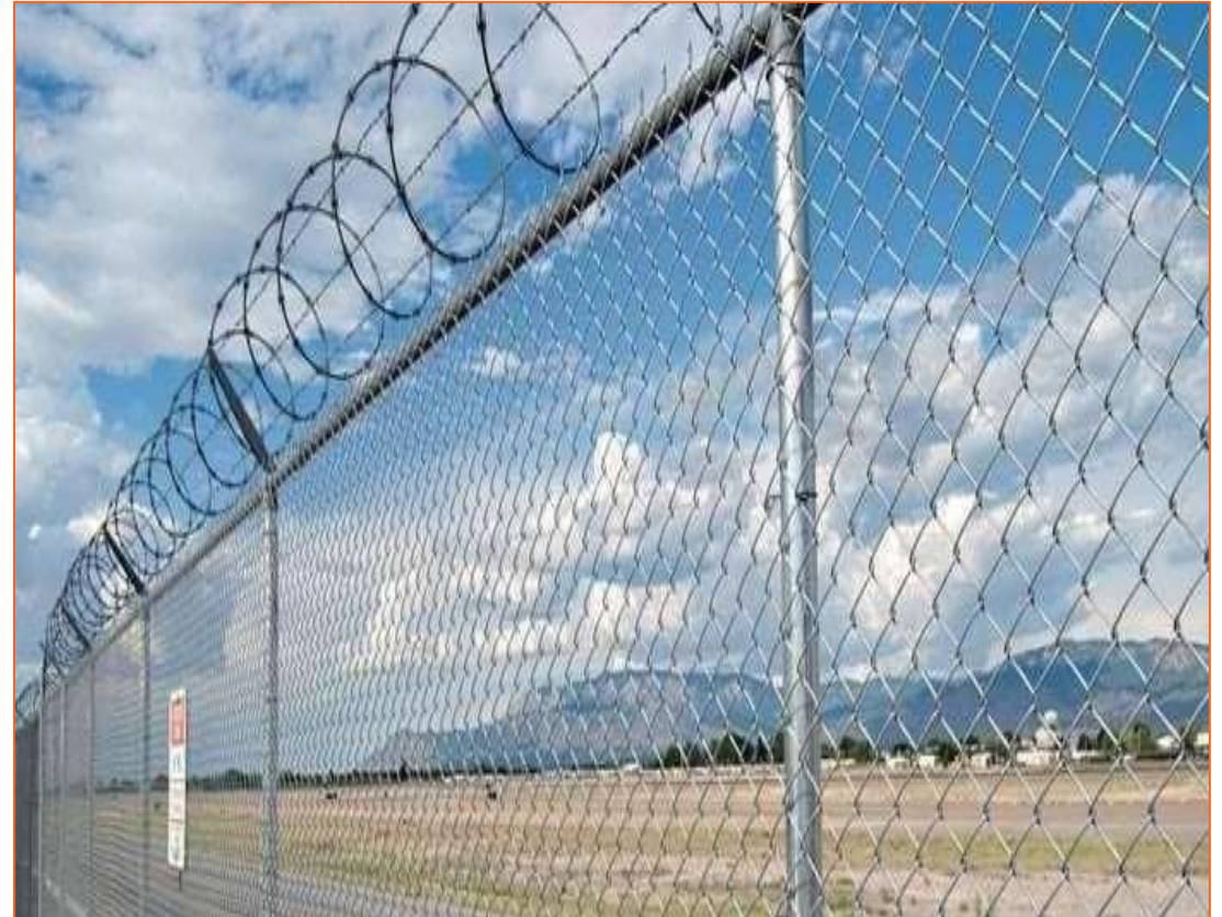
Chain Link Fence
